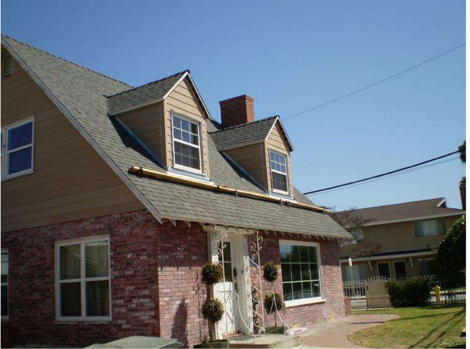
Finished Downey Roof and Siding
